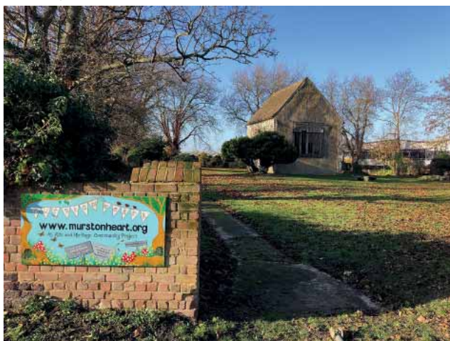
Murston Old Church – a Scheduled Monument with the project to repair and re-use the church supported by the Council.
