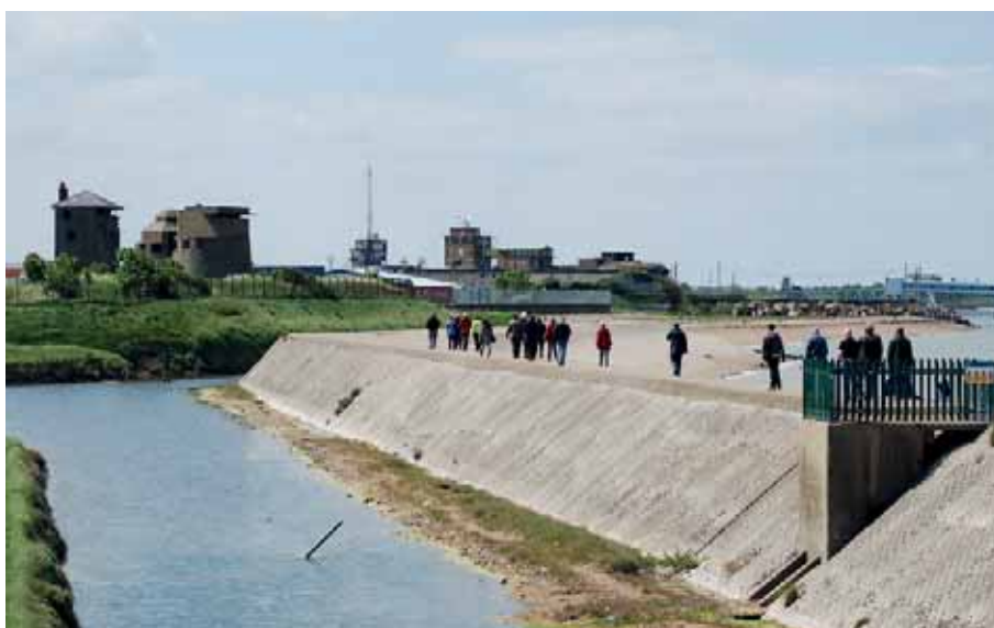
First World War Gun Emplacement at Sheerness – located within moated (scheduled) Sheerness Defences structure. Image provided courtesy of Simon Mason.
