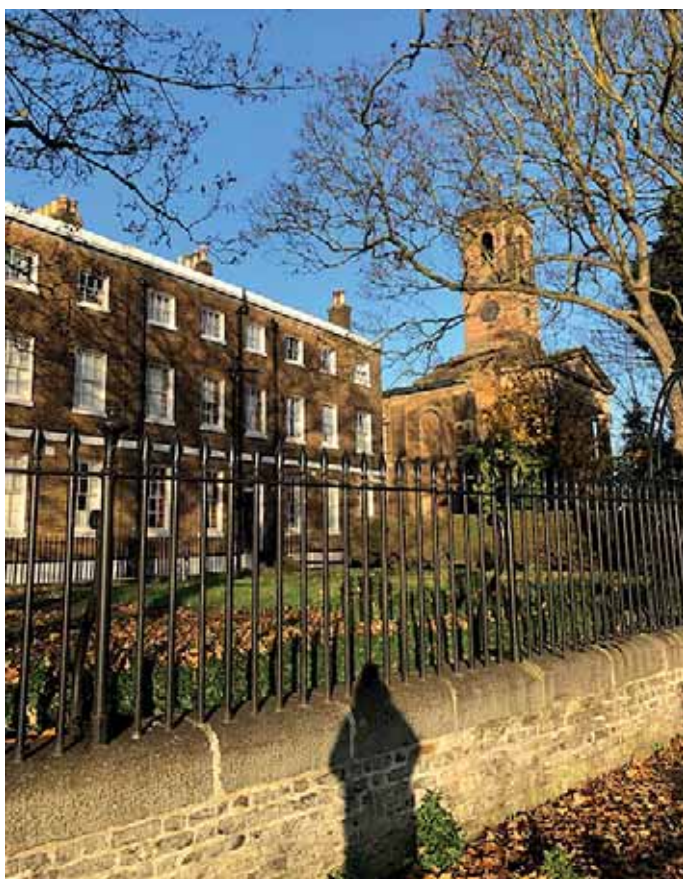
The grade II* listed Naval Terrace and Dockyard Church, Sheerness.
